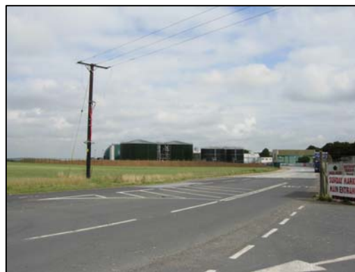
Existing AD facility
